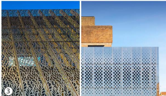
③ Roof mounted plant with decorative screening to conceal plant from view
